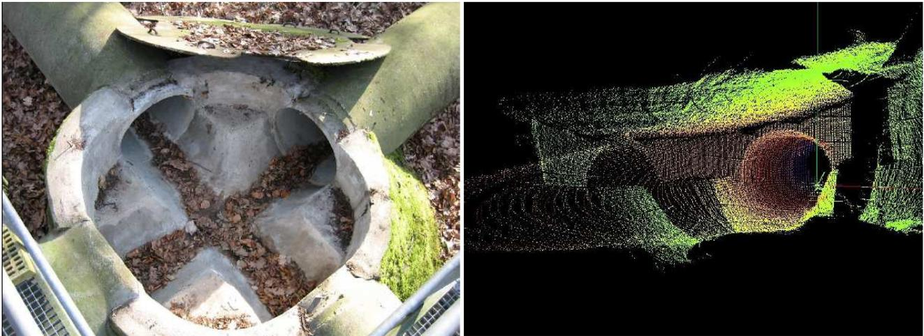
Figure 5: Left: A jointed part of two sewers at Fraunhofer Campus Birlinghoven. Right: Scanning result displayed by 3D viewer.
